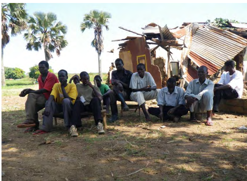
Residents of Lukodi sitting next to a dilapidated house in the trading centre. Reconstruction and recovery has been slow in many areas because most of the infrastructure was destroyed during the conflict. Photo Credit: Roza Freriks
